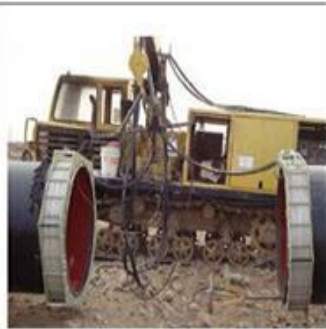
Flexible air-cooled inductor cable.
